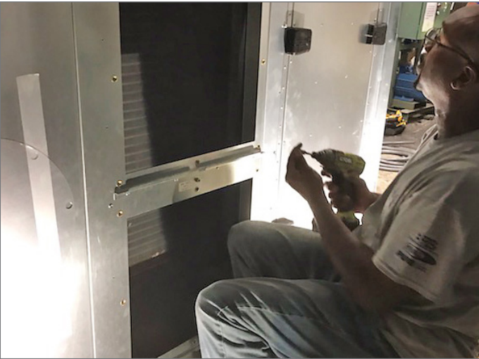
Q-PAC Fan Wall Installation
