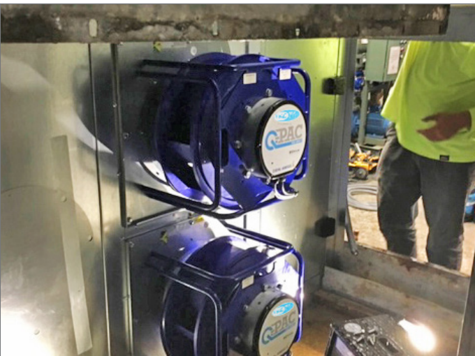
Q-PAC Fan Installation
