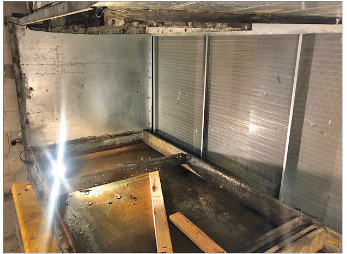
AHU Interior Prep
