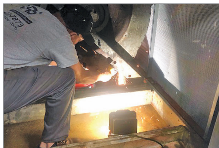
Old Blower Removal
