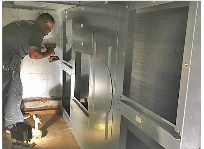
Q-PAC Fan Wall Installation
