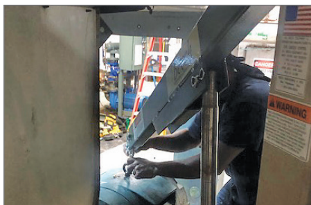
Old VFD Blower Motor Removal
