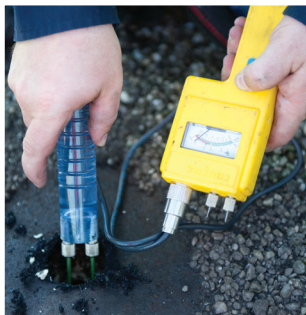
MOISTURE PROBE TESTING
